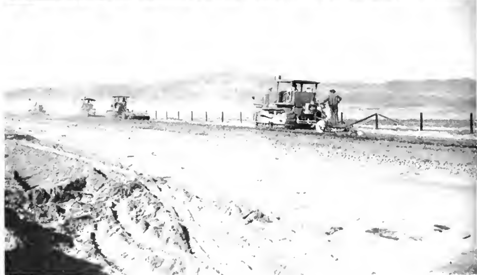
UPPER—Cement treatment in 1937. Bagged cement spotted along grade is ready for spreading on this pioneer project by state forces. LOWER—Teams of tractors tow farm plows to mix in-place material and cement.
